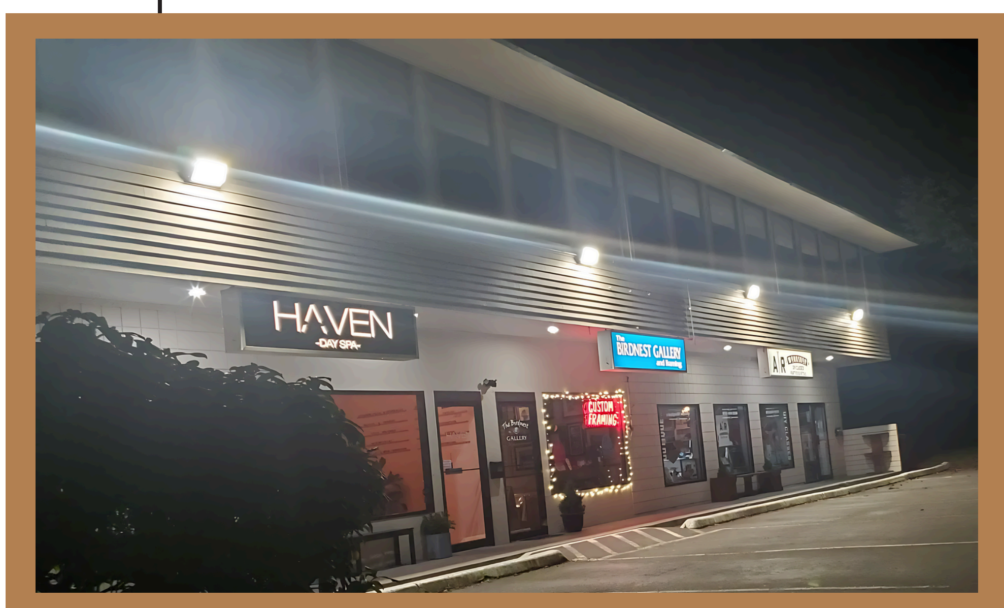
PHOTO OF COMPLETED LIGHTING AT DUSK
